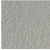
Zinc Rocktop Structure
